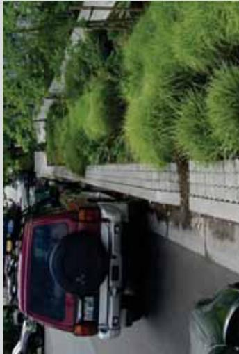
Curb side: width of compacted shoulder is 24" +/-; Shoulder has weed cover of less than 25%; Less than 20% of paver joints contain weeds
