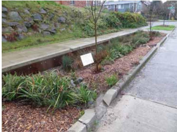
*Photo on left is an access lid over a deep infiltration facility (UIC screen well). Photo on the right is for a bioretention cell facility with horizontal pit drain, structural soil cells below the sidewalk and perforated corten steel wall along the sidewalk side of the facility.*
