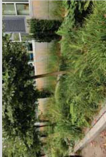
Curb side: width of compacted shoulder is less than 12"; vegetation growing in the road shoulder or plants overhanging into the shoulder more than 12"; More than 20% of paver joints contain weeds
