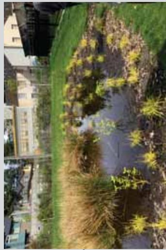
Soils appear compressed and ponding observed 72+ hours following rain period
