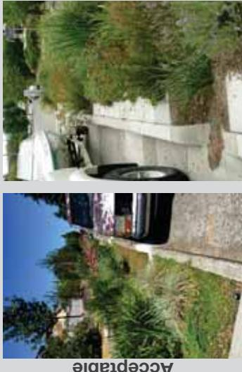
Curb side: width of compacted shoulder is 24" +/-; Shoulder has weed cover of less than 25%; Minor debris in curb inlet
