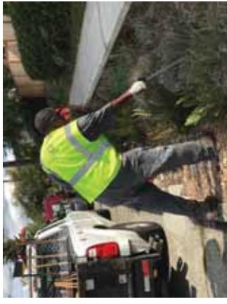
The most important times to remove debris and trash from the bioretention cell are before and after a storm. Heavy rains can cause trash and debris to collect around curb openings and overflow drains and block stormwater flow.
