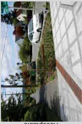
Moderate trash, debris and sediment at trench drain grates
