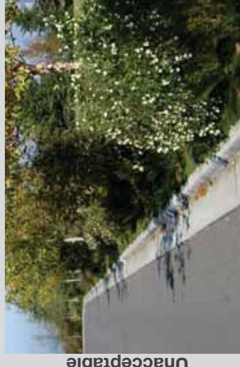
Curb side: width of compacted shoulder is less than 12"; vegetation growing in the road shoulder or plants overhanging into the shoulder more than 12"
