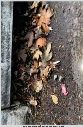
Heavy trash, debris and sediment plugging trench drain grates
