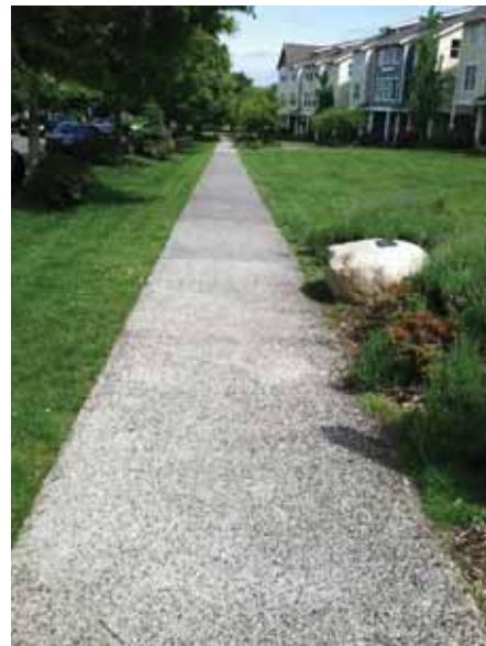
*Photo on left is a pervious concrete path between bioretention cells for access between public sidewalk and curb. Photo on right is public pervious concrete sidewalk.*
