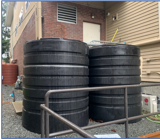
Two out of the four 856-gallon cisterns.
